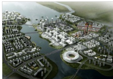
Urban planning's role in resource utilization will only continue to grow in importance. - arch.nus.edu.sg
