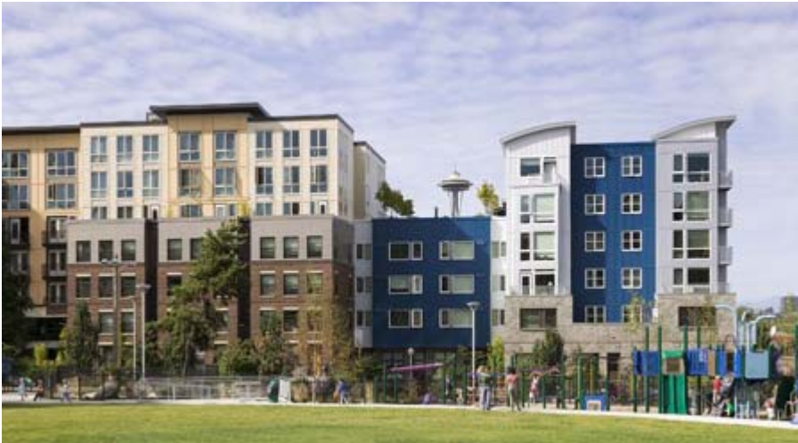
Residents in the transit-oriented Alcyone development can easily walk to Cascade Park or hop on a bus to downtown Seattle. Steven Keating, Courtesy Vulcan.
